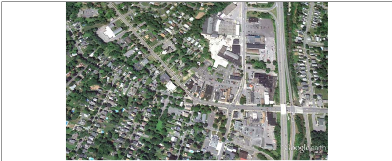
Figure 3: Aerial photography of the relocated Sauquoit Creek and Sauquoit Valley Expressway in New Hartford, a suburb of Utica. Source: Google Earth Pro
